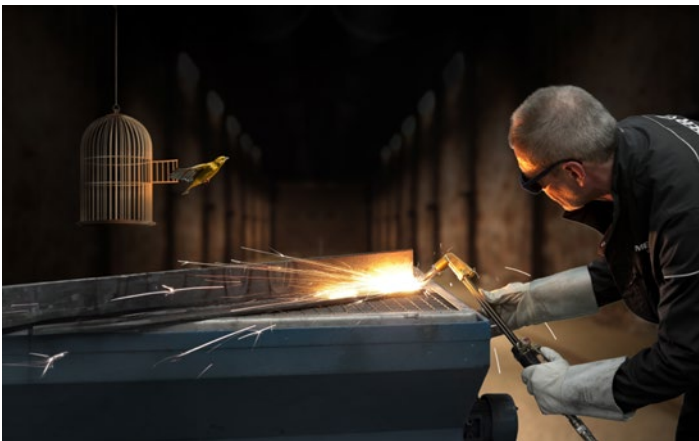
Photo 2: If there is a leak, the new S.A.T. safety system stops the gas flow automatically and the flame is extinguished.
